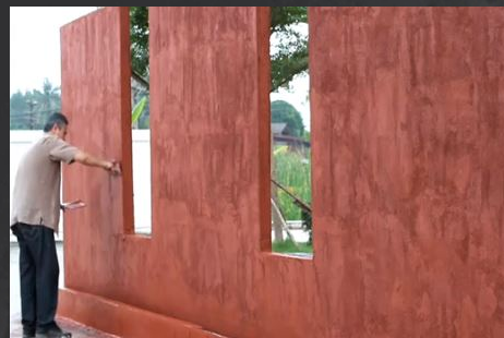
Cement base coat is rendered
