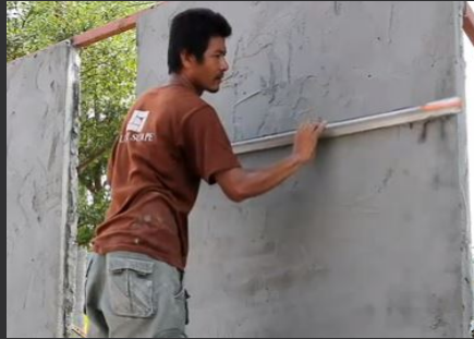
Cement base coat is rendered
