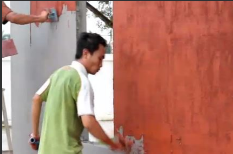
Cement base coat is rendered
